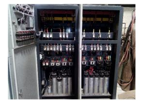
Figure 2.19: Inside of a PFI plant.
