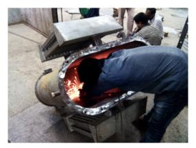
Figure 2.14: Welding the tank.
