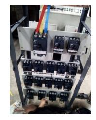
**Figure 2.4:** *Circuit breakers and other components getting installed.*
