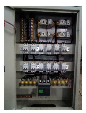
Figure 2.21: Inside a typical DB.
