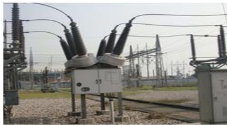
Figure 4-10: SF6 circuit breaker
