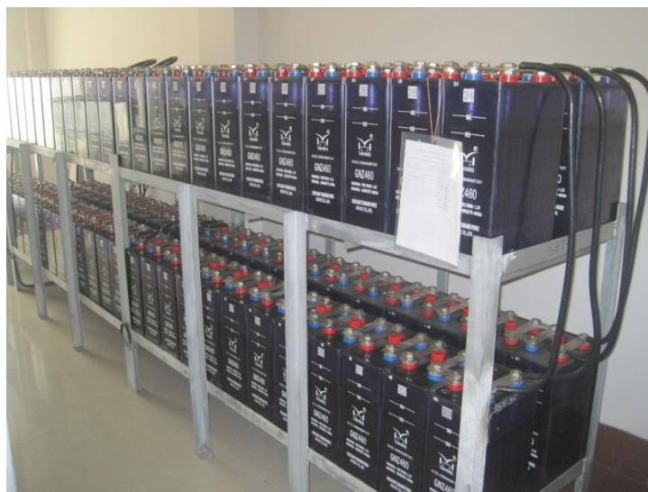
Fig-4.4: Series connected Nickel Cadmium battery
