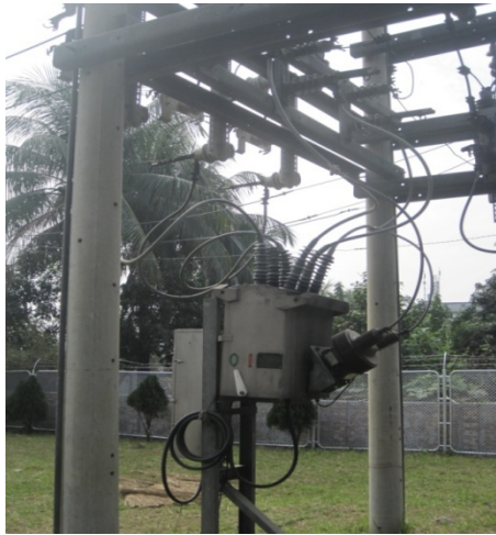
Fig4.15: An ACR (auto circuit recloser)
