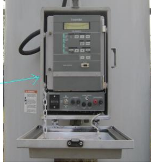
Fig4.14: manually setup part of AVR
