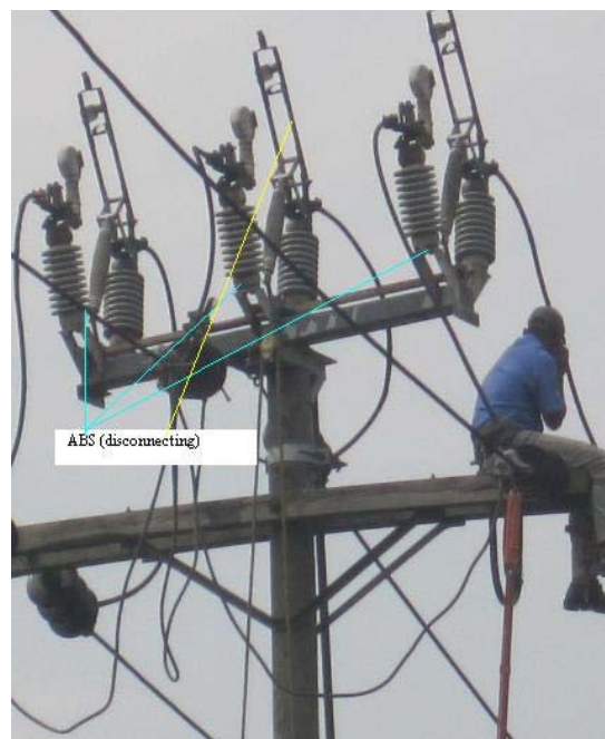
Fig4.12: Manually operate an ABS (disconnected)
