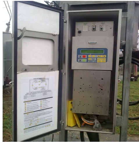
Fig4.16: Internal setup box of ACR
