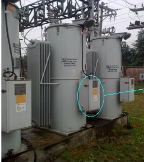
Fig4.13: Auto voltage regulator
