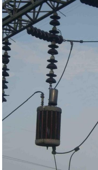
Figure 4.19: Wave Trap in APSCL.
