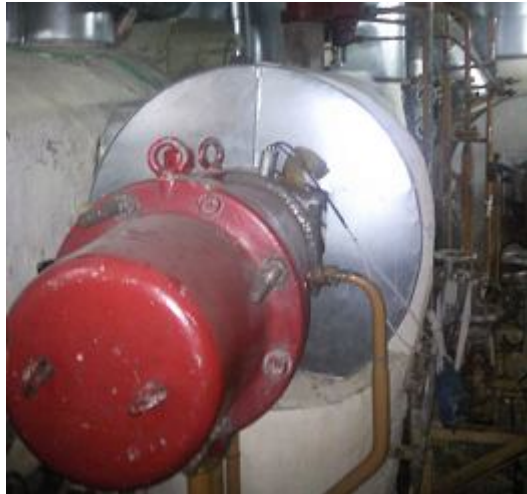
Figure 5.12: Shut-off valve of turbine (Unit 3).
