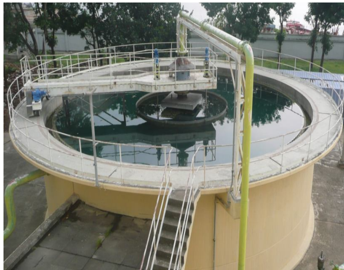
Figure 2.3: Water Filter House
