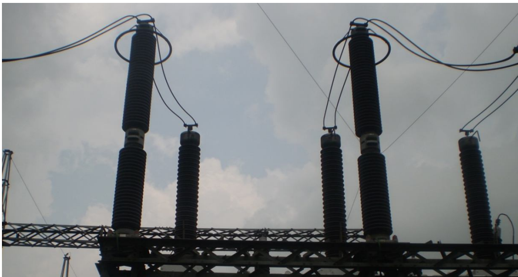
Figure 4.15: Metal Oxide arrester in APSCCL.
