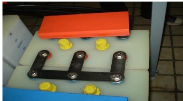
Figure 11: Series connection of batteries.
