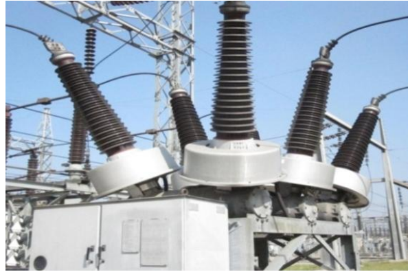
Figure 30: Oil circuit breaker.
