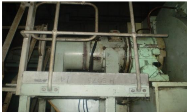
Figure 3: Brushless thyristor exciter used in CCPP.
