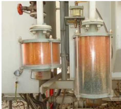
Figure 4.5: Silica Gel Breather
