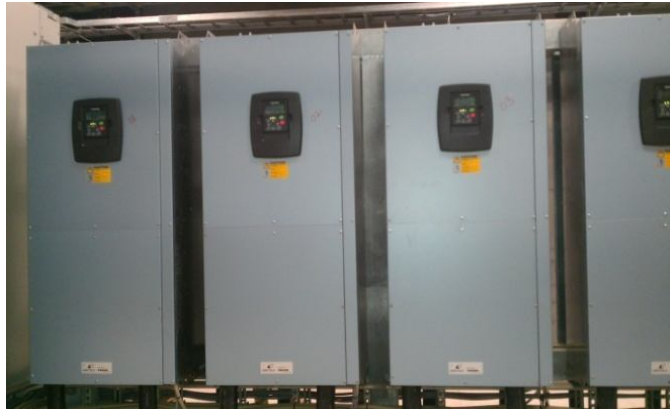
Figure 2.20: Frequency converter
