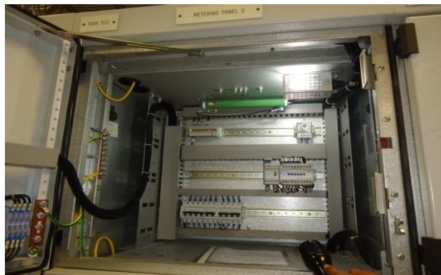
Figure 2.17: Metering panel
