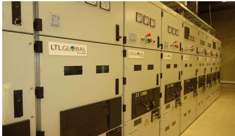
Figure 2.15: MV switchgear
