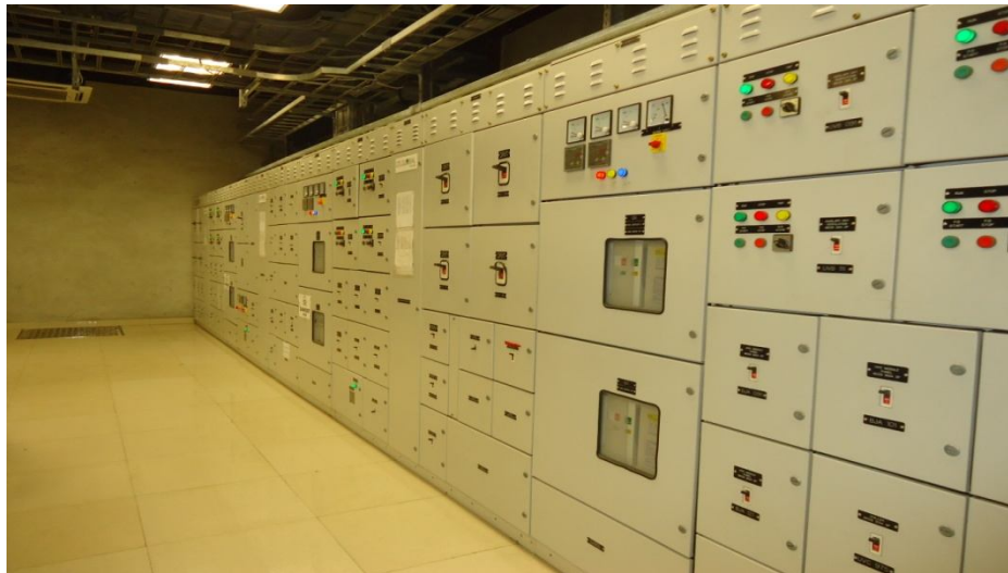
Figure 2.14: LV switchgear
