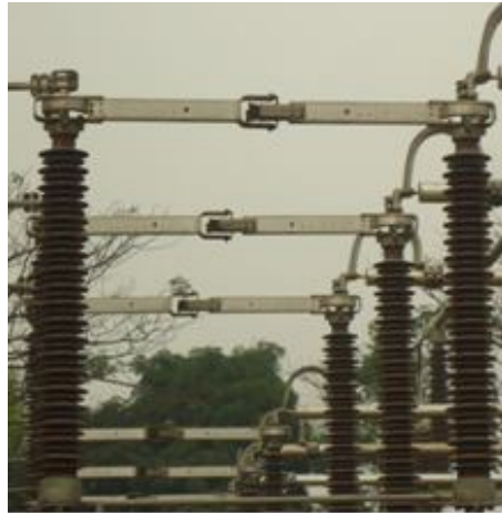
Figure 4.14: Isolator used in DBPAL
