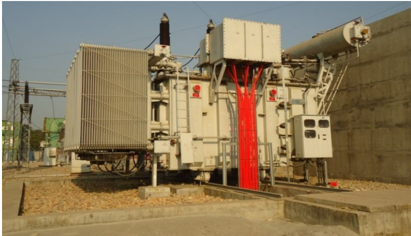
Figure 4.1: Liquid Immersed Transformer used in Dutch Bangla Power and Associates Limited (DBAPL)
