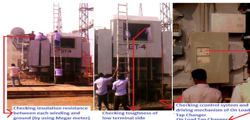
Figure 3.3: Transformer maintenances at Uttara grid-substation.
