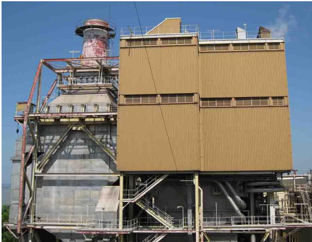
Figure 7.1: Thermal power plant.
