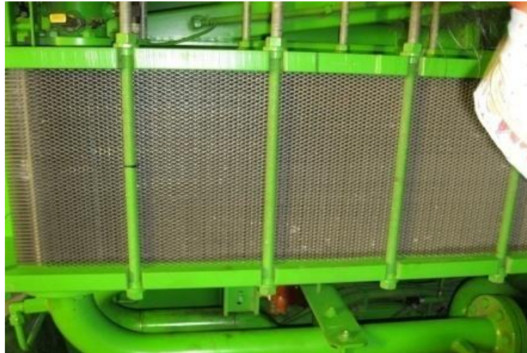
Figure 2.3: Air suction from atmosphere of a gas engine.
