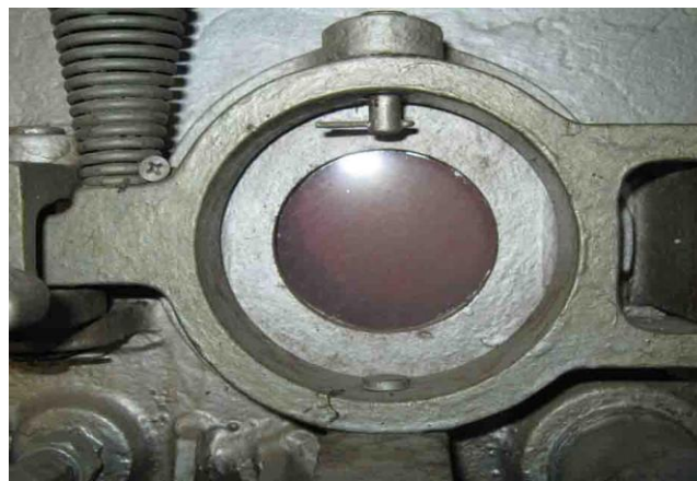
Figure 7.2: Burner view glass.
