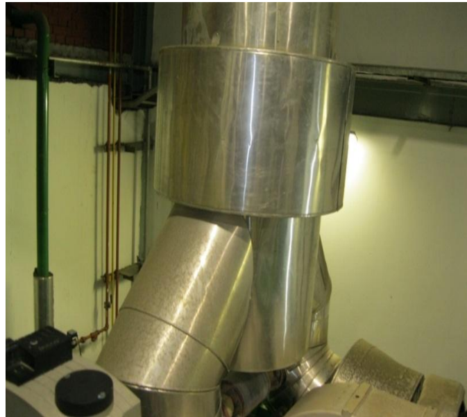
Figure 2.5: Gas exhaust path inside the engine room.
