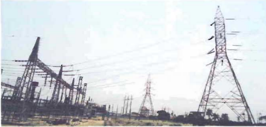
Figure 54: Transmission Line (overhead line) in APSCL
