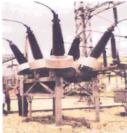
Figure 3.14: SF6 circuit breaker
