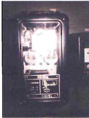
Figure 3.8: Reverse power relay
