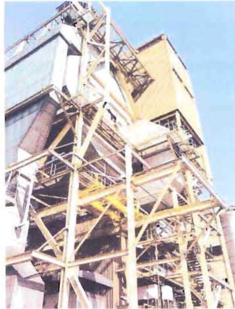
Figure 2.16: Water tube boiler used in APSCL
