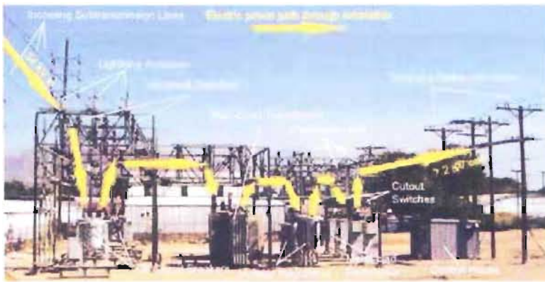
Figure 4.1: Substation
