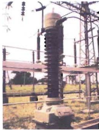
Figure 4.13: Potential Transformer
