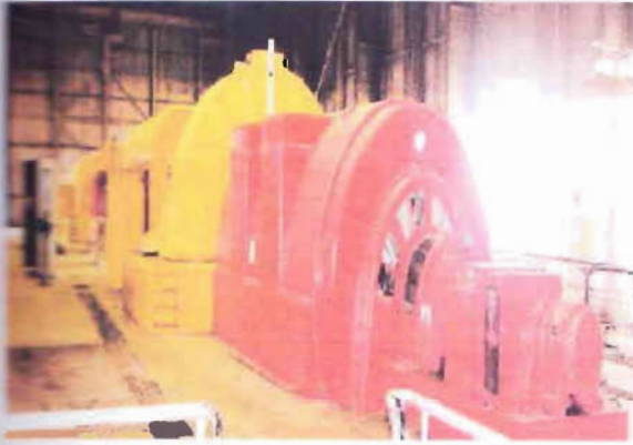
Figure 2.2: AC generator of ST-2 and GT-1 of APSCL
