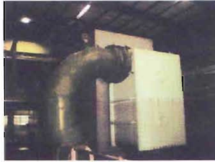
Figure 2.31: Condenser used in steam turbine section of combined cycle power plant
