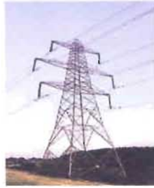
Figure 4.18: Transmission line & Tower
