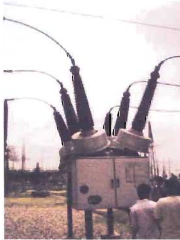
Figure 4.8: SF6 Circuit Breaker
