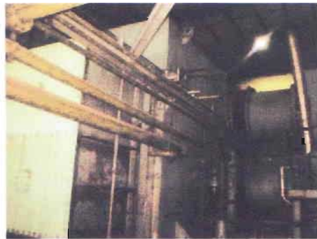
Figure 2.26: Centrifugal compressor used in APSCL [11]
