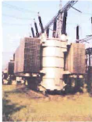
Figure 4.11: Step-up transformer
