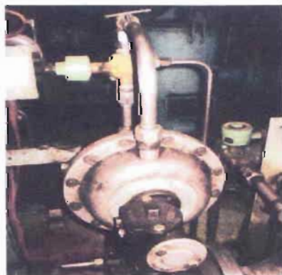
Figure 2.33: Pneumatic valve
