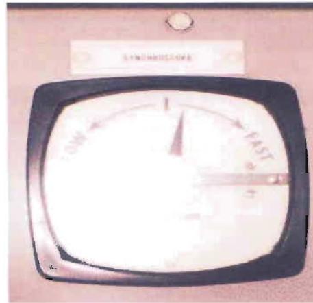
Figure 2.11: Synchroscope
