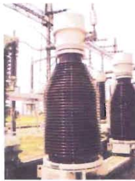
Figure 4.12: Current Transformer
