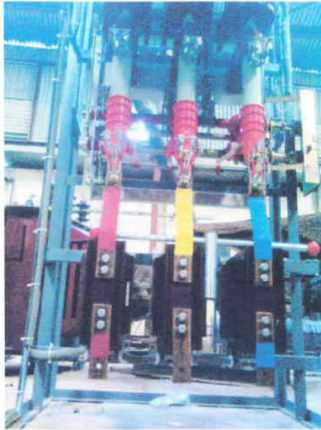
Figure 7.2: Load Break Switch (LBS)
