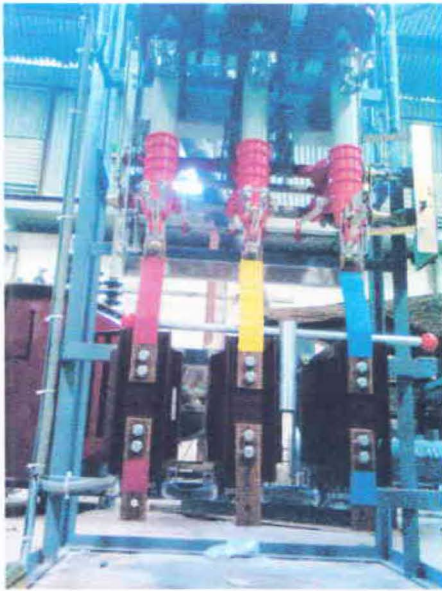
Figure 6.4: Inside of HT Switchgear
