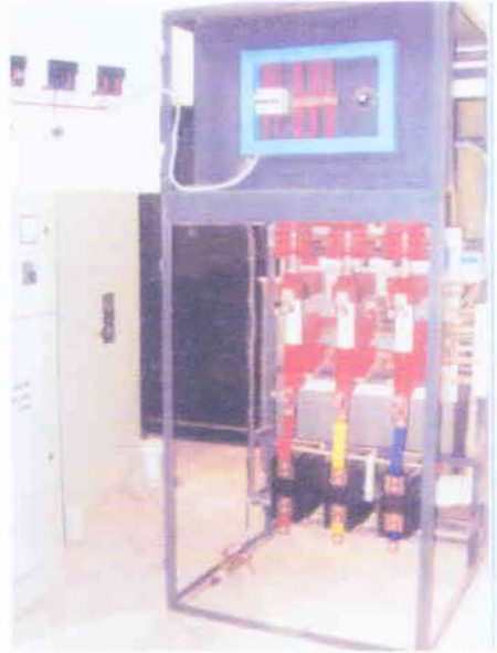
Figure 6.4: Inside of HT Switchgear
