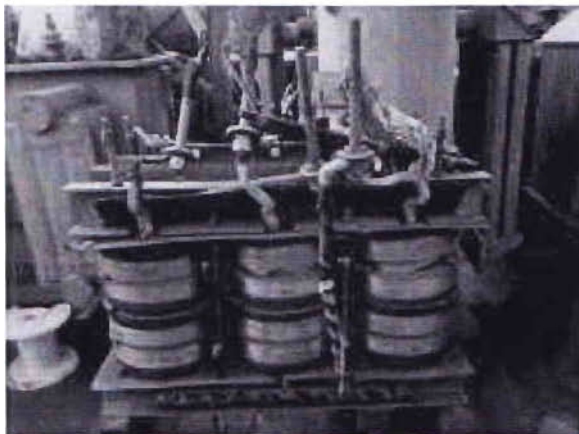
Figure 3.4.2: Rewinding transformer coil
