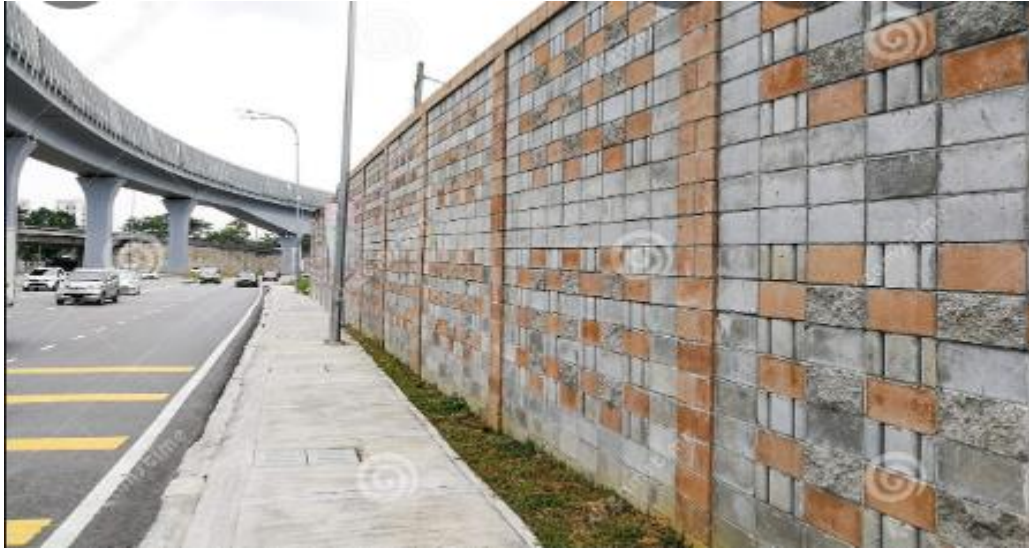
Figure 8.13 Brick wall barrier
