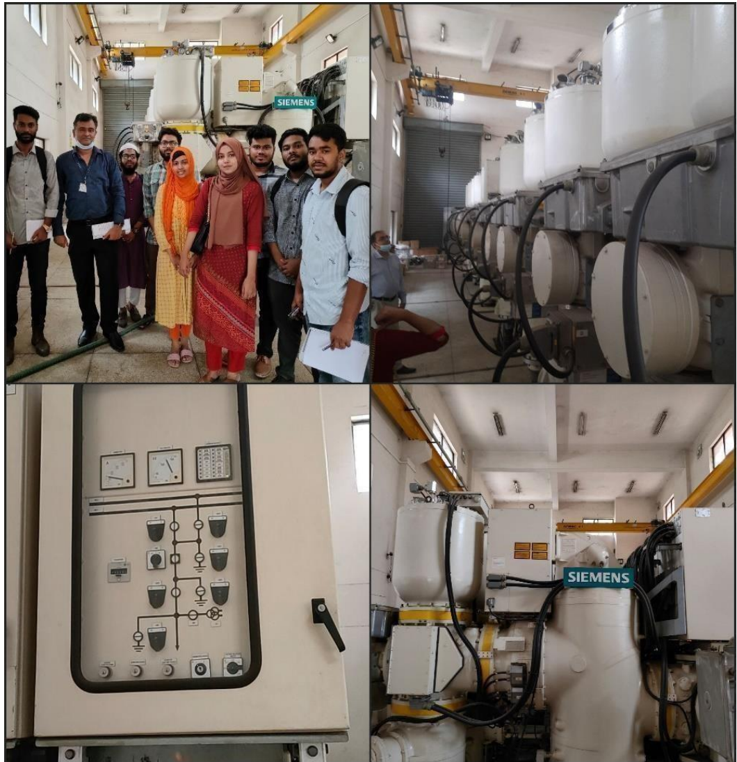
Figure -Dhanmondi Sub-Station
