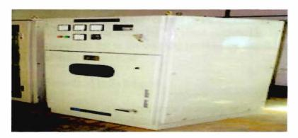
Fig 23: Load Break Switch. [7]
