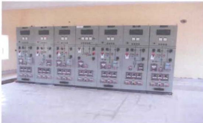
Figure 4.3: Programmable logic control (PLC) unit of UPGD
