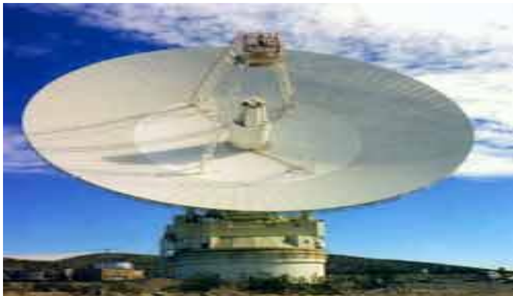
Figure1.8: A typical parabolic reflector antenna
