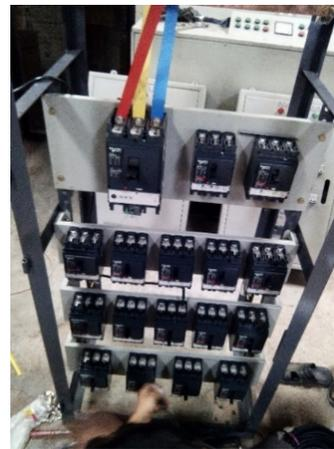
**Figure 2.4:** *Circuit breakers and other components getting installed.*
