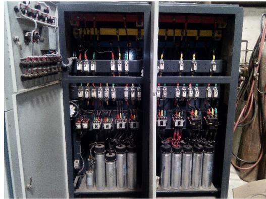
**Figure 2.19:** Inside of a PFI plant.
