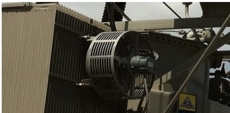
Figure 4.8: Cooling fan in transformer [11].
