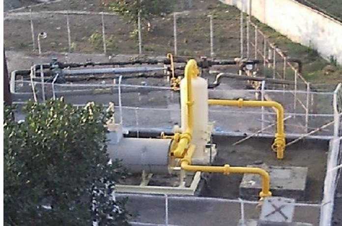
Figure 2.5: Fuel system of combined cycle power plant [11].
