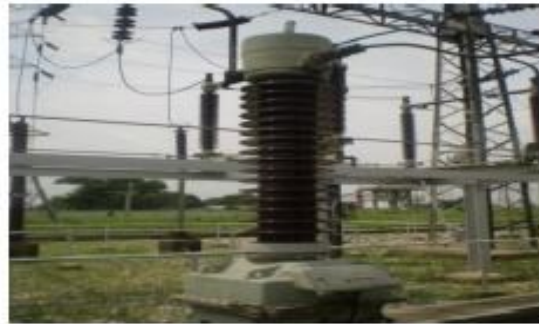
Figure 4.4: Potential transformer [11].
