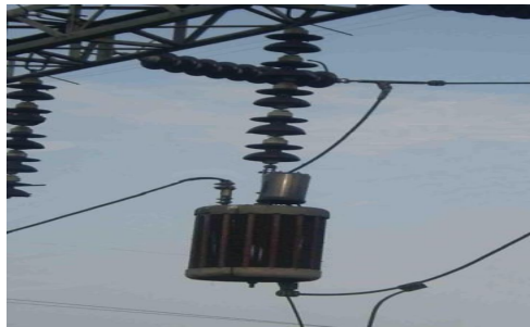
Figure 4.9: Wave trapper at APSCL [11].
