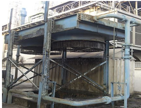
Figure 2.6: Lube Oil cooling plant [11].
