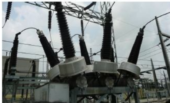
Figure 4.6: Circuit Breaker [11].
