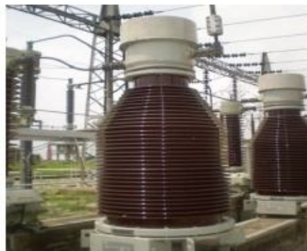
Figure 4.3: Current transformer [11].
