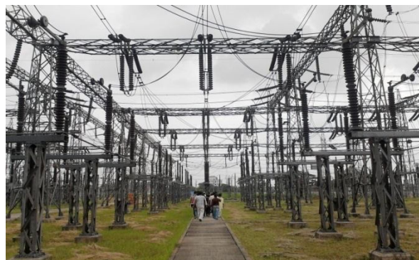
Figure 4.5: The system of bus-bars in APSCL [11].
