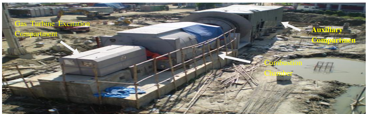
Figure 3.1: Generator Unit at the setup time of Siddhirganj 2 X 120 MW PPP
