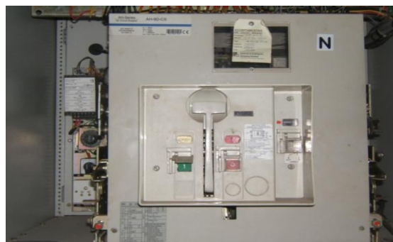
Figure 4.2: Air Circuit Breaker used in EGCB
