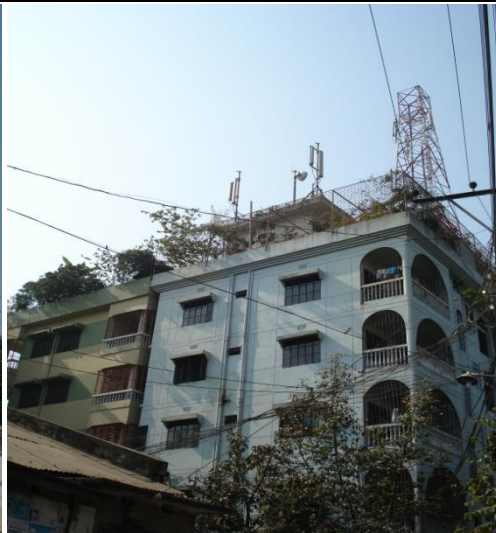
Figure 2.8.2: Roof Top Site
