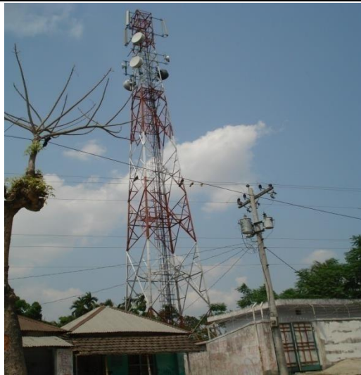
Figure 2.8.1: Green Field Site
