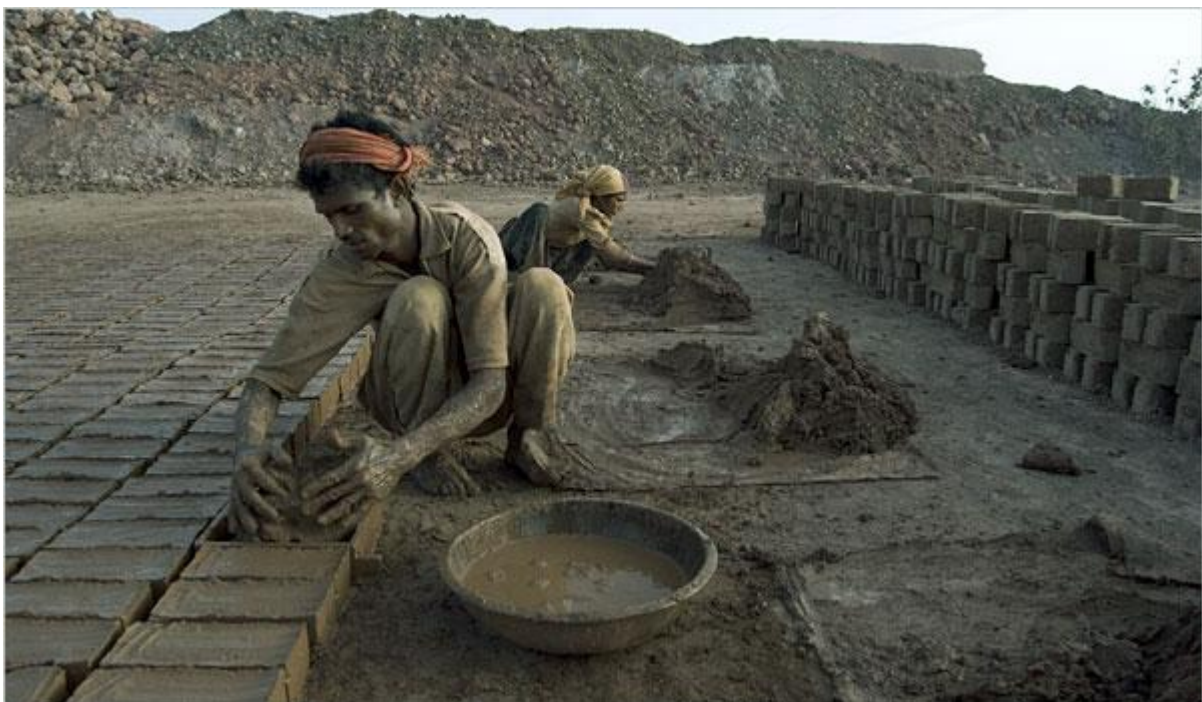
Fig.3: Molding in brick making process
