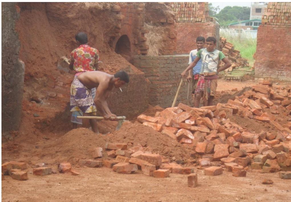
Fig.6: Workers preparing trench in heating area of a brick field
