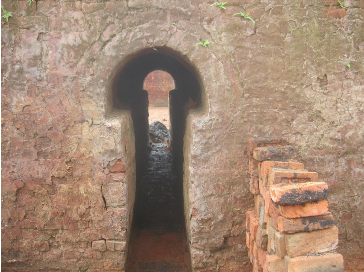
Fig.4: Firing Chamber for brick making
