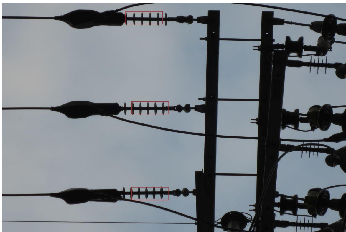
Figure 3.23: Applying non-maximum suppression, correctly able to reduce the number of bounding boxes
