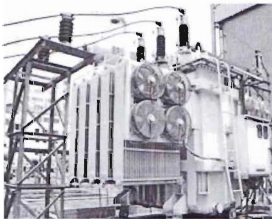
Fig 4.12: Cooling system
