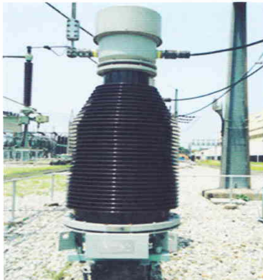
Figure 4.3: A single phase, oil immersed 132 KV current transformer of APSCL
