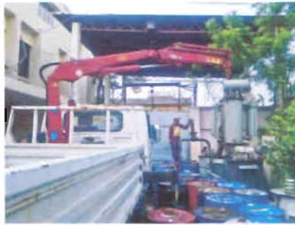
Figure 3.11: New transformer is being lifted to truck by crane.
