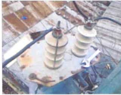
Figure 3.6: H.T side testing in progress
