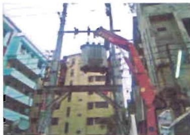
Figure 3.12: A new transformer was being lifted up by crane .
