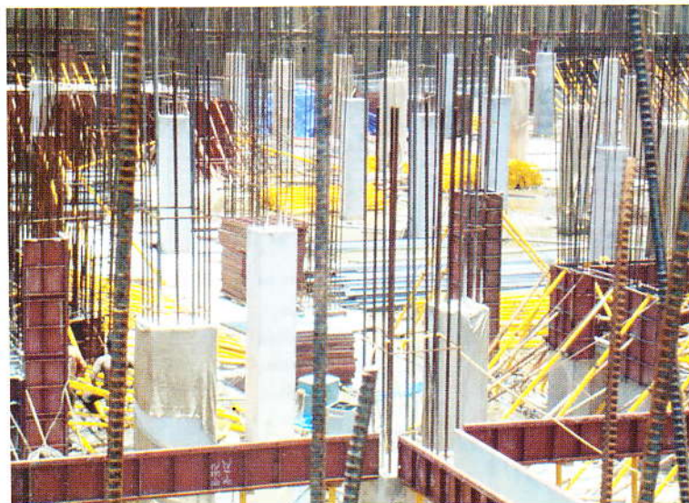
EWU's own campus construction work in progress
