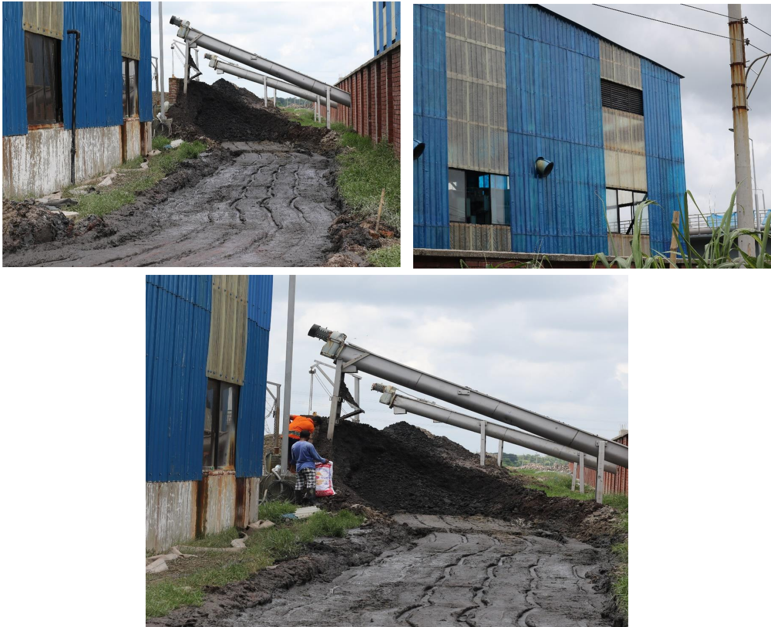
Figure 3.4: Damp Zones of Tannery Common Effluent Treatment Plant Sludge (CETPS)
