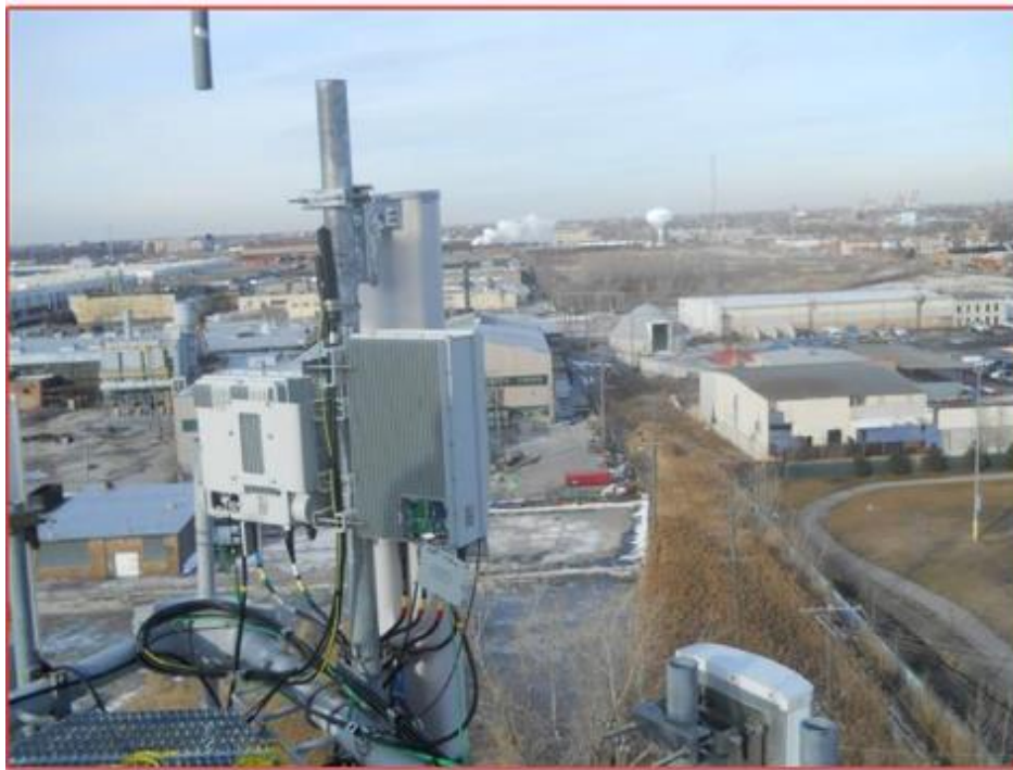
Figure 10: Router of RF Mesh
