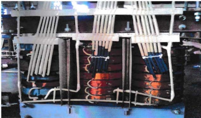
Figure 26: Delta connection
