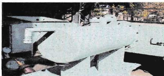
Figure 13: Transformer's Conservator
