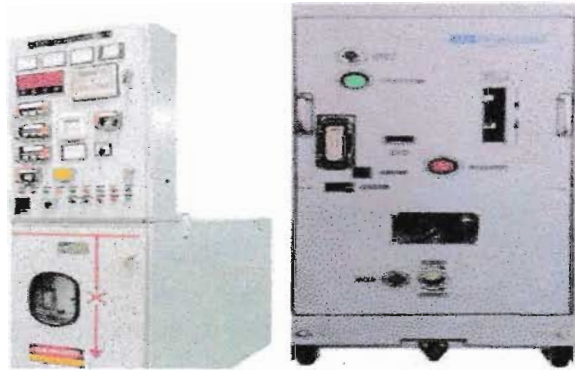
Figure 27: Outdoor and indoor type VCB
