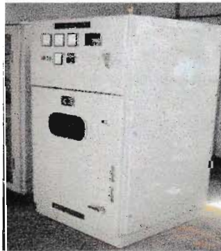
Figure 29: Load Break Switch
