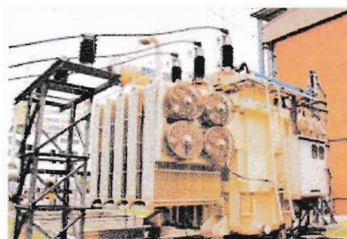
Figure 1: 33/11KV Transformer
