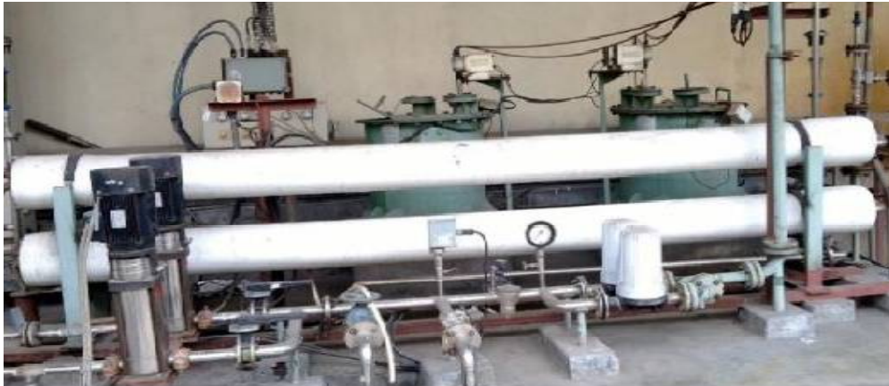
Figure 2.3: Water treatment plant [2]
