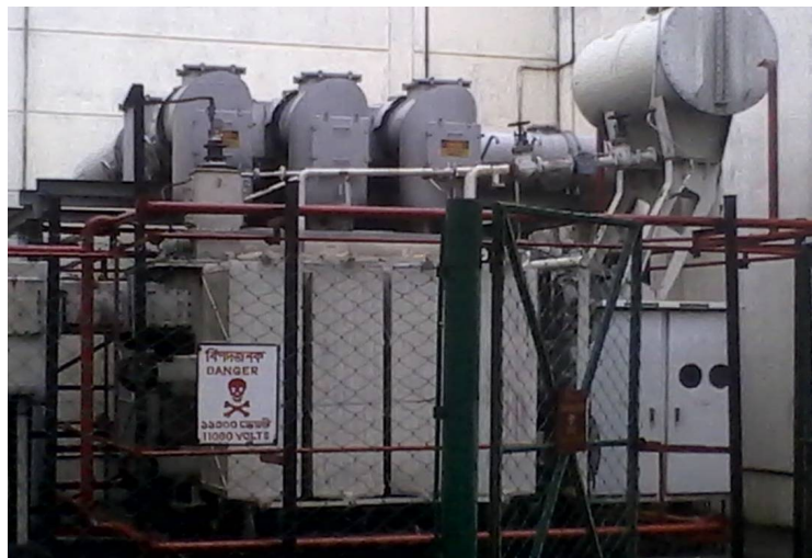
Figure 3.2: Medium voltage unit auxiliary transformer [2]
