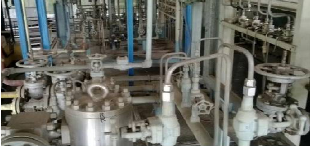
Figure 2.4: Lubricating oil system [2]
