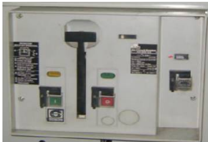
Figure 5.1: Air circuit breaker [2]
