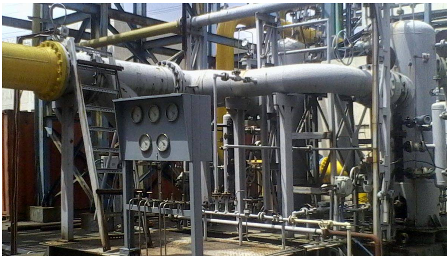
Figure 2.1: Gas filter system [2]
