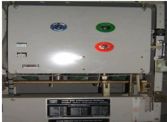
Figure 5.3: Vacuum circuit breaker [2]
