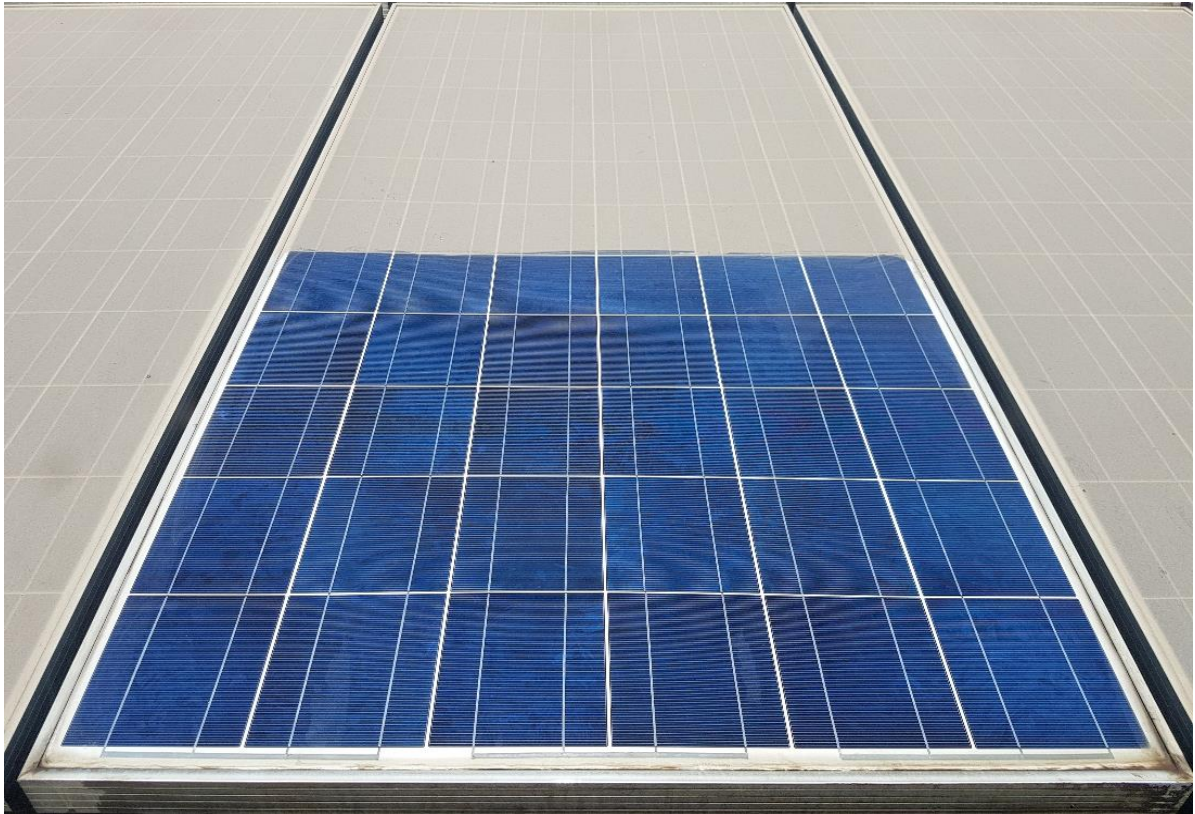
Figure 4.10: Solar panel after cleaning.
